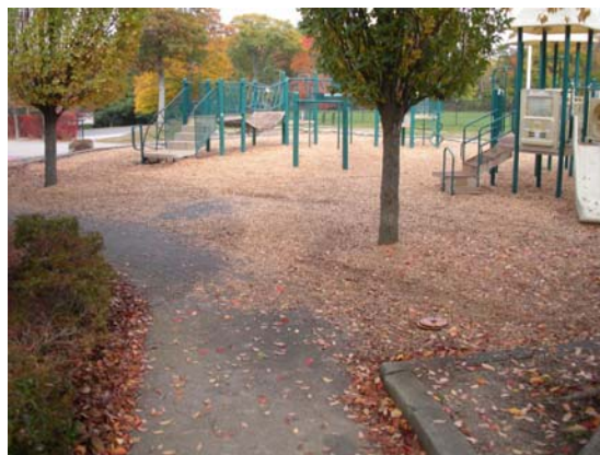
LACK OF ACCESSIBLE PATHS TO PLAY STRUCTURES
