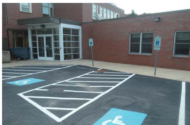
LACK OF CURBING, WHEELSTOPS AND BOLLARDS AT NORTHEAST ENTRANCE
