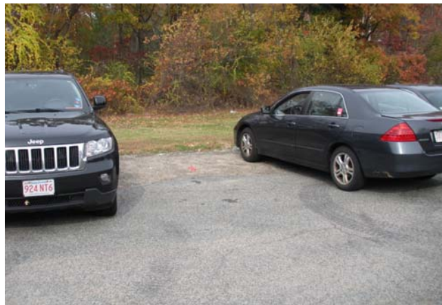
GRAVEL EXTENSION OF PARKING AREA WITH NO CURBING
