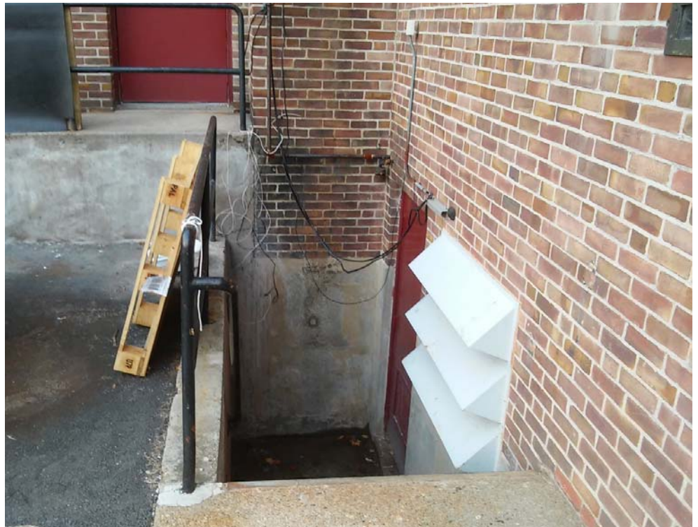
HANGING WIRES AND STANDING WATER AT BOTTOM OF LOWER LEVEL EGRESS
