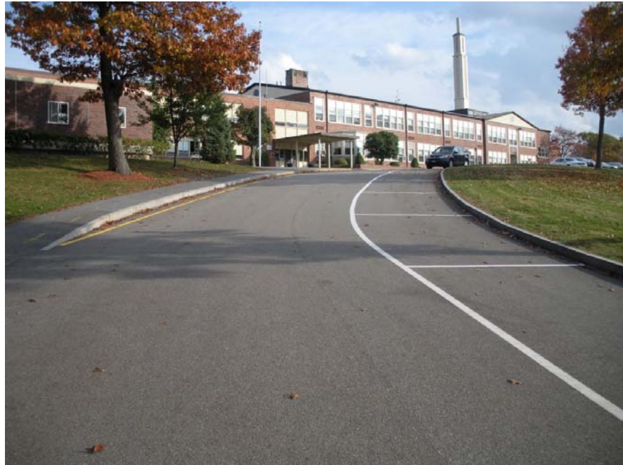
WALKWAY ALONG FRONT BUS/PARKING LOOP THAT EXCEEDS MAAB SLOPE REQUIREMENTS
