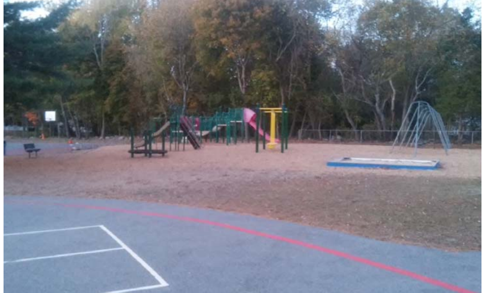
NO ACCESSIBLE ROUTES PROVIDED TO THE WOOD-FIBER PLAY AREA AND STRUCTURES
