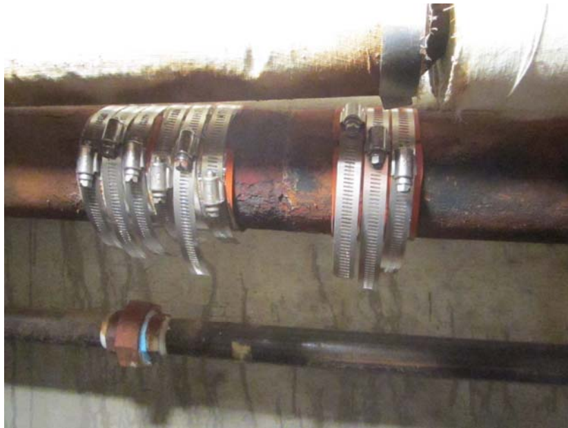
PATCHED STEAM PIPING. THE SMALLER DIAMETER CONDENSATE PIPE HAS BEEN REPLACED TO THE RIGHT OF THE UNION (JOINT).
