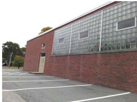
BRICK AND GLASS BLOCK REPOINTING REQUIRED
