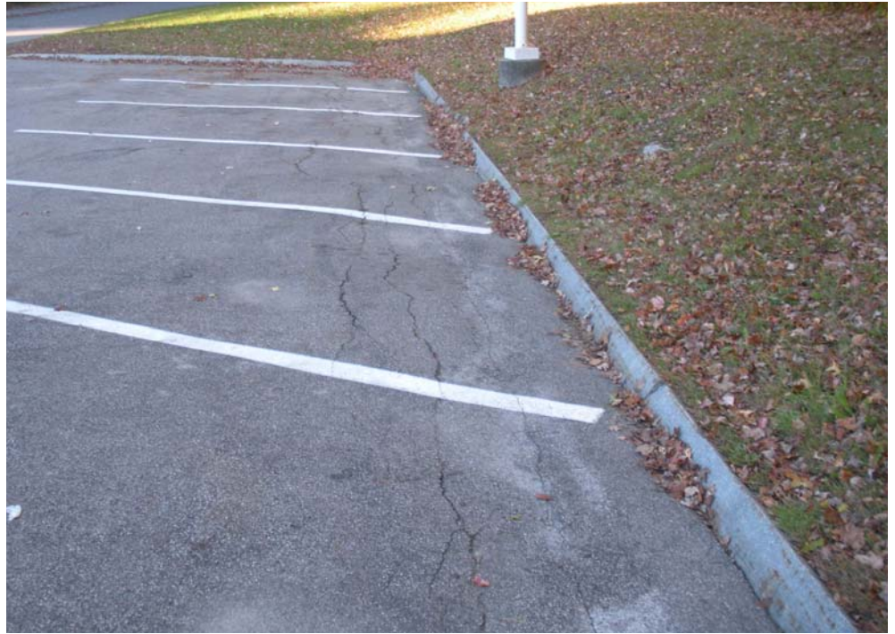
FATIGUE CRACKING AND SETTLEMENT ALONG EDGE OF EAST PARKING LOT
