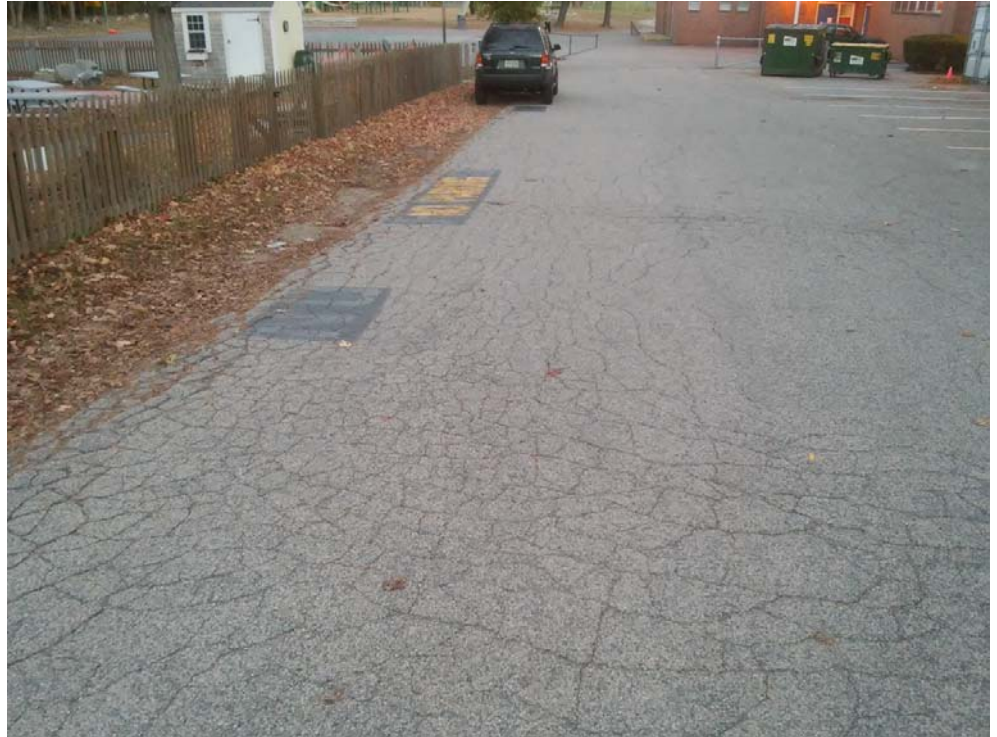
FATIGUE CRACKING IN NORTHWEST PARKING AREA/ACCESS DRIVE
