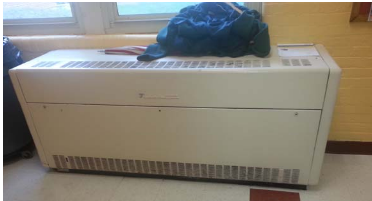
ORIGINAL HERMAN NELSON UNIT VENTILATOR
