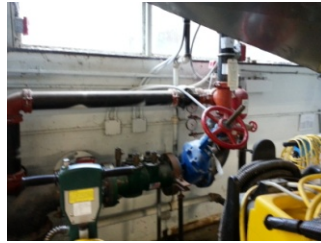
FIRE PROT. PIC 1
