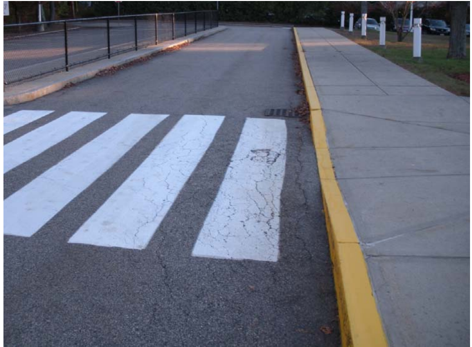
LACK OF DETECTABLE WARNING PANEL AT BUS LOOP CURB CUT, AND PAVEMENT CRACKING
