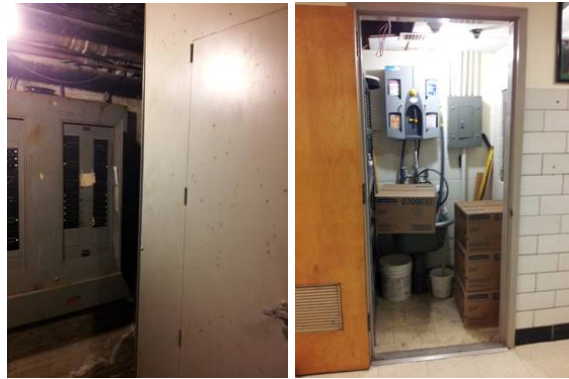
FIG 1: POWER DISTRIBUTION PANELS
