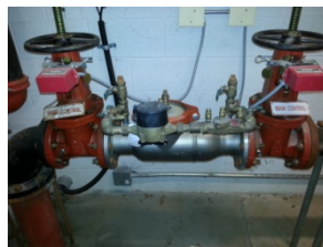
FIRE PROT. PIC 2
