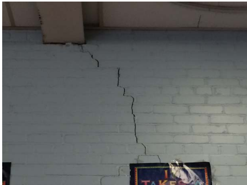
THE ORIGINAL LOAD BEARING BRICK WALLS IN THE ART ROOM (FORMERLY AND AUDITORIUM STAGE), ARE CRACKED BELOW WHERE A STEEL ROOF GIRDER BEARS ON THEM AT EACH END.
