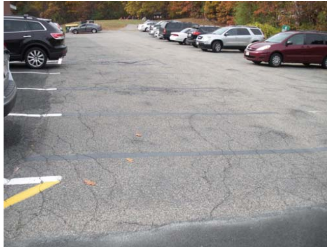
FATIGUE CRACKING AND HEAVING/SETTLEMENT IN NORTH PARKING LOT
