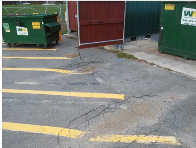
PAVEMENT RUTTING AT DUMPSTER AREA
