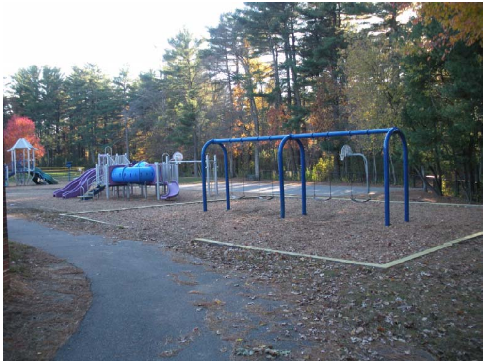
LACK OF ACCESSIBLE PATHS TO PLAY STRUCTURES
