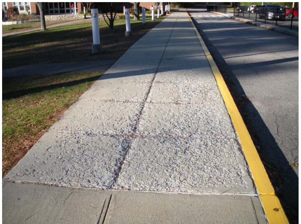
CONCRETE DETERIORATION AT WALKWAY ADJACENT TO BUS LANE
