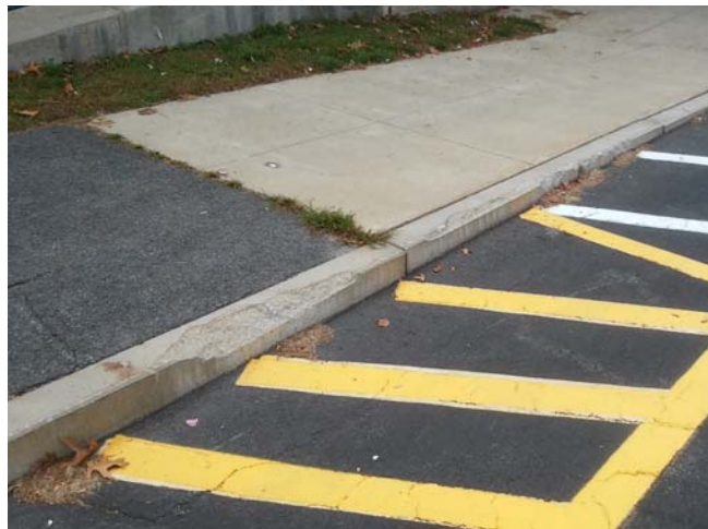
CONCRETE CURB DAMAGE/DETERIORATION NEAR NORTHEAST ENTRANCE
