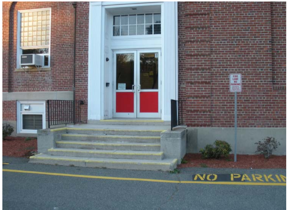
NON-ACCESSIBLE FRONT ENTRANCE AND NON-COMPLIANT HANDRAILS
