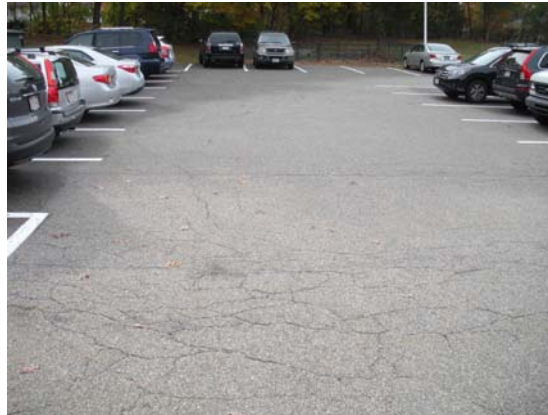
FATIGUE AND BLOCK CRACKING IN SOUTH PARKING LOT
