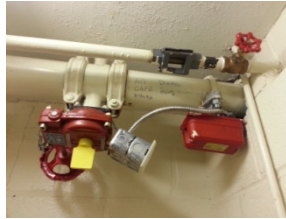
FIRE PROT. PIC 1
