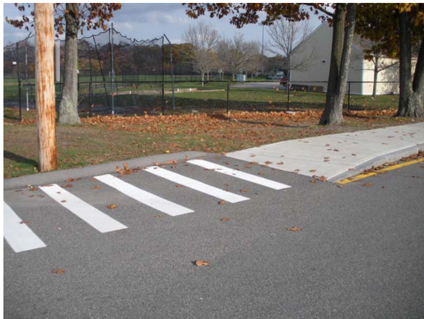
CURB RAMP LACKING DETECTABLE WARNING STRIP AT INTERSECTION OF FRONT BUS LOOP AND PARENT QUEUE LOOP
