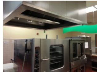
FIRE PROT. PIC 4
