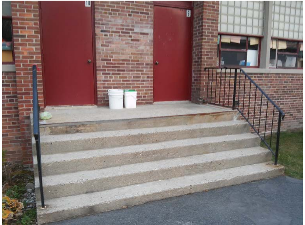
NON-ACCESSIBLE BUILDING EGRESS POINT ON WEST SIDE OF BUILDING
