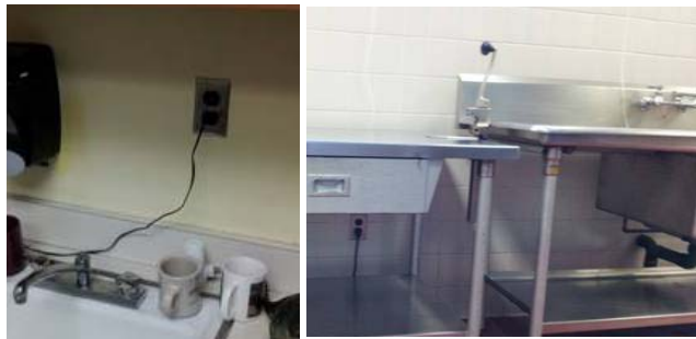
FIG 3: RECEPTACLES NEAR SINKS
