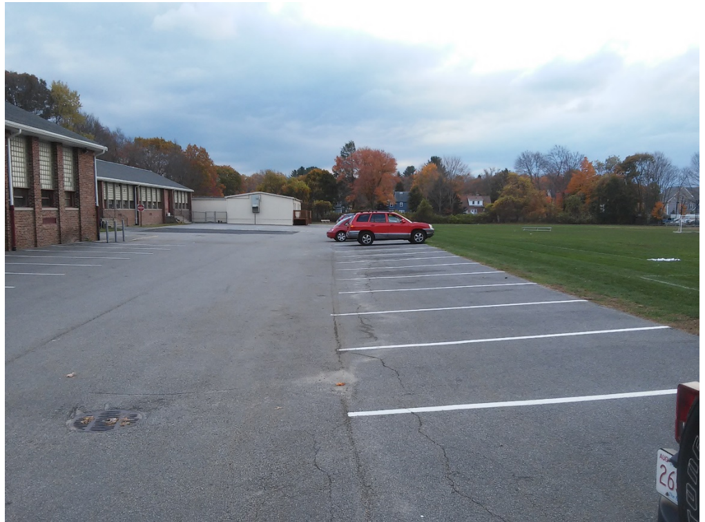
SEAM AND LONGITUDINAL CRACKING IN WEST PARKING LOT
