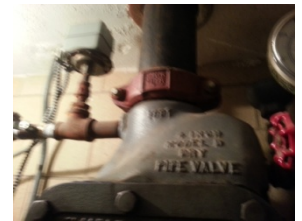
FIRE PROT. PIC 8
