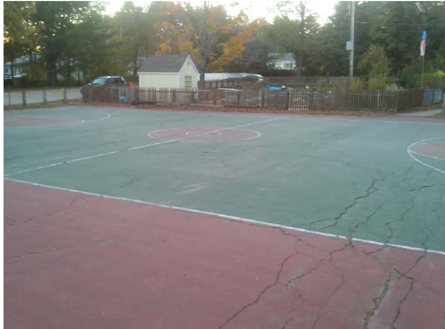
FATIGUE AND TRANSVERSE CRACKING AT BASKETBALL COURTS
