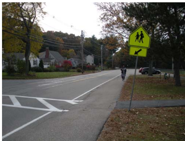
LACK OF DETECTABLE WARNING PANEL AT CURB CUT ONTO GAY STREET
