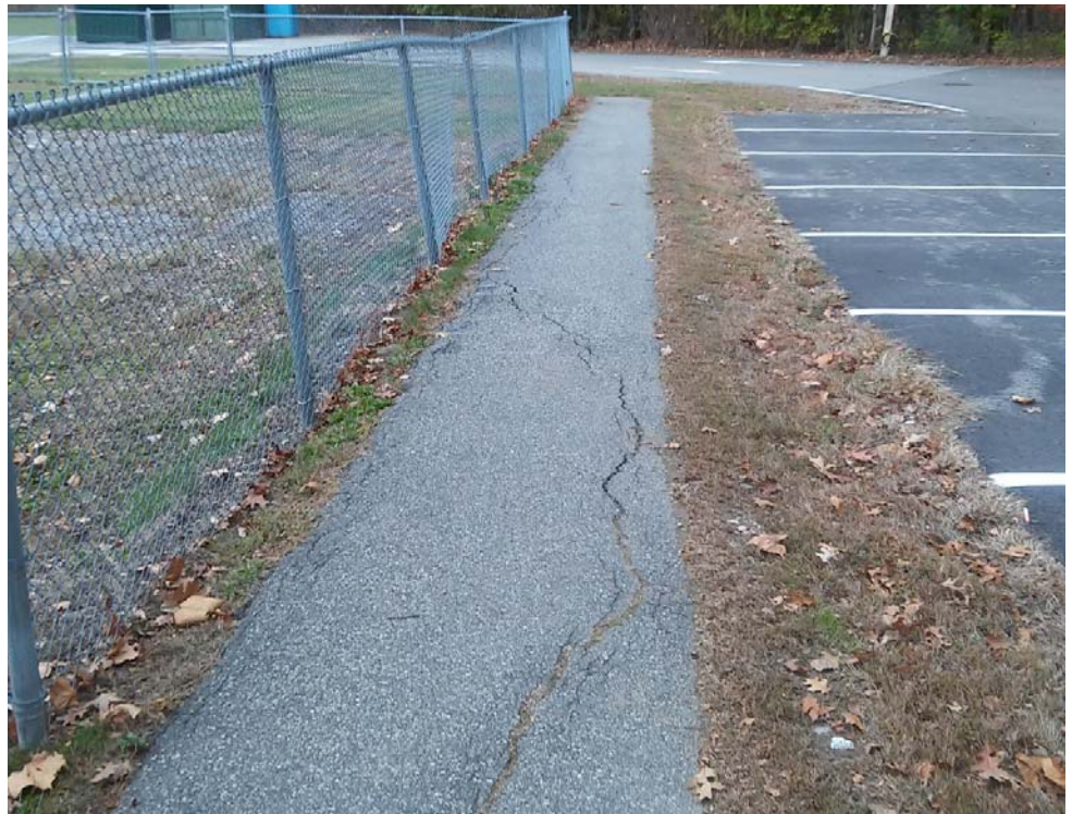
CRACKING AND HEAVING IN WALKWAY ADJACENT TO NORTHERN PARKING AREA
