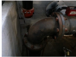
FIRE PROT. PIC 3
