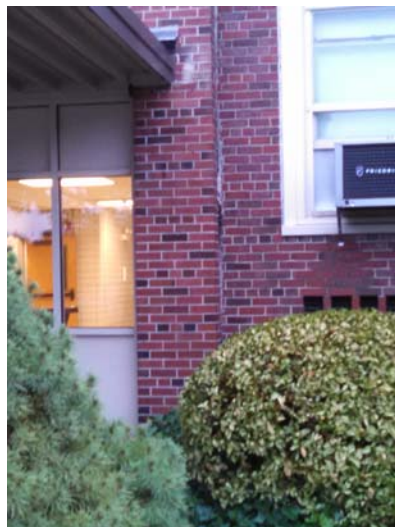
REPOINT BRICKS AT MAIN ENTRY
