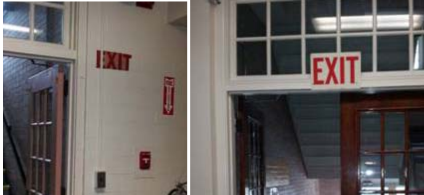
FIG 2: EXISTING EXIT SIGNS
