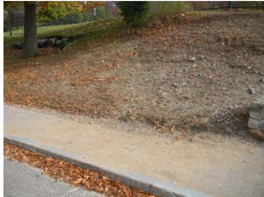
EROSION OF STEEP SLOPE ADJACENT TO PLAYFIELDS
