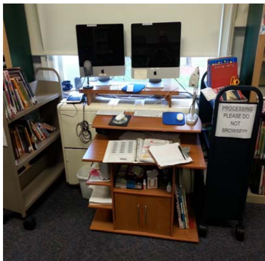
MEDIA CENTER UNIT VENTILATOR. UVs ARE TYPICALLY NEARLY OBSCURED WITH FURNITURE, STACKED TEXTBOOKS AND OTHER TEACHING RESOURCES.
