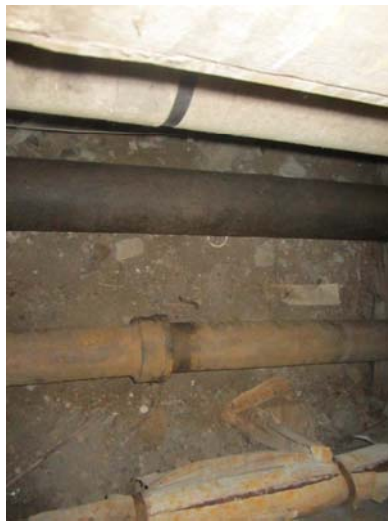
LOOKING DOWN INTO THE STEAM TUNNEL FROM A CLASSROOM HATCH. NOTICE THE DAMAGED ASBESTOS PIPE INSULATION AND DEBRIS ON THE FLOOR.
