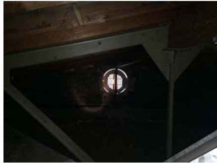
ATTIC LOUVER LEAK
