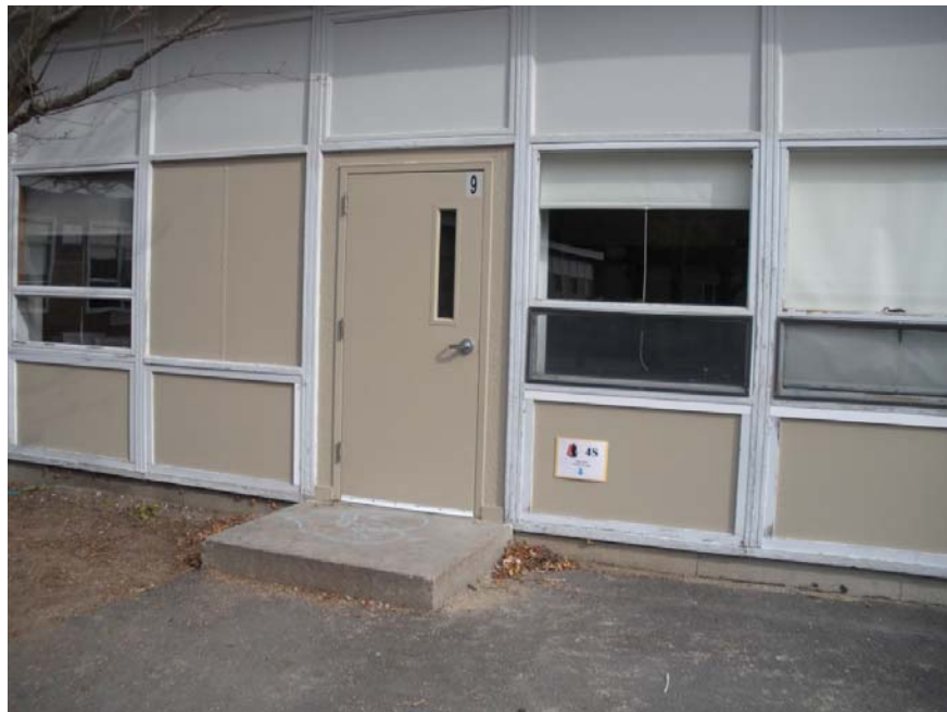
NON-ACCESSIBLE BUILDING EGRESS ON SOUTH SIDE OF BUILDING
