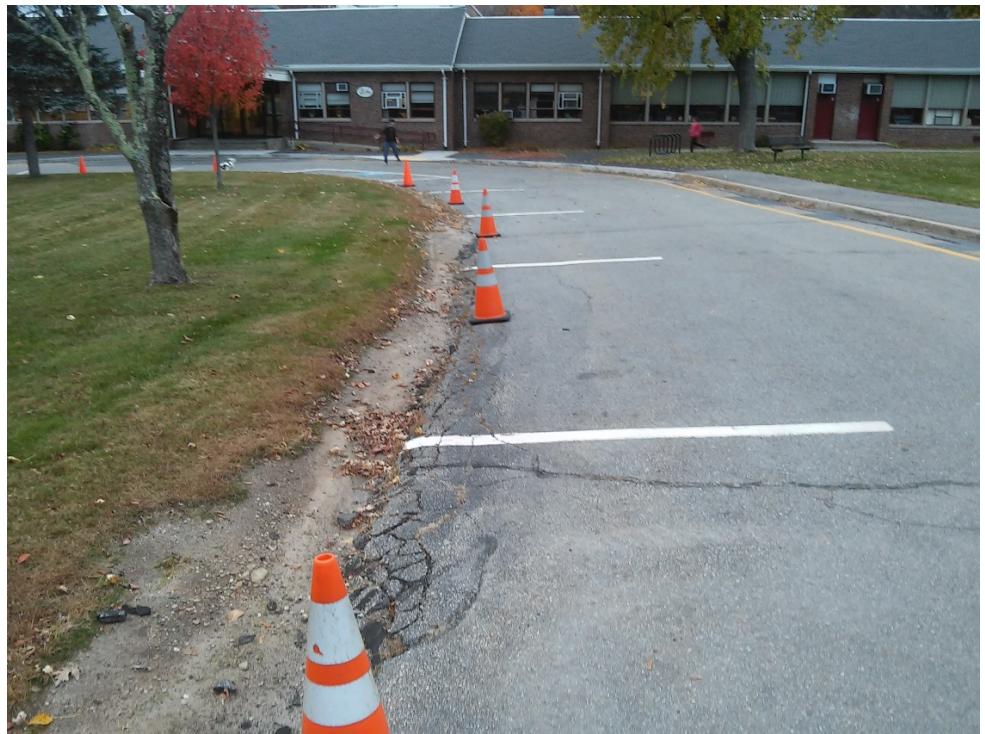
EDGE CRACKING AND ADJACENT RUTTING IN LANDSCAPE AREA AT FRONT BUS LOOP/PARKING AREA
