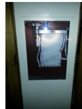
FIRE PROT. PIC 7
