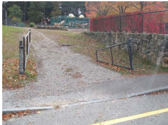
ERODED GRAVEL ACCESS PATH TO GRASS PLAYFIELDS; LACK OF DETECTABLE WARNING PANELS
