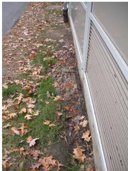
STANDING WATER ALONG BACK (WEST) SIDE OF BUILDING
