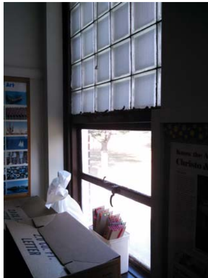
RUSTING STEEL FRAME WINDOWS IN GLASS BLOCK
