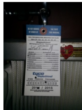
FIRE PROT. PIC 6
