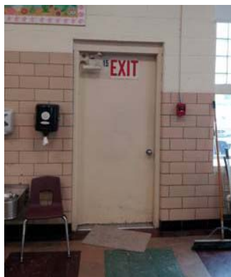
FIG 2: PRINTED EXIT SIGN
