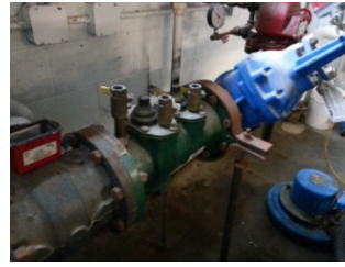
FIRE PROT. PIC 2
