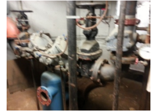
FIRE PROT. PIC 4
