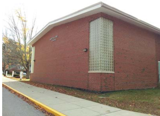
A FEW HAIRLINE CRACKS IN GLASS BLOCK MORTAR JOINTS
