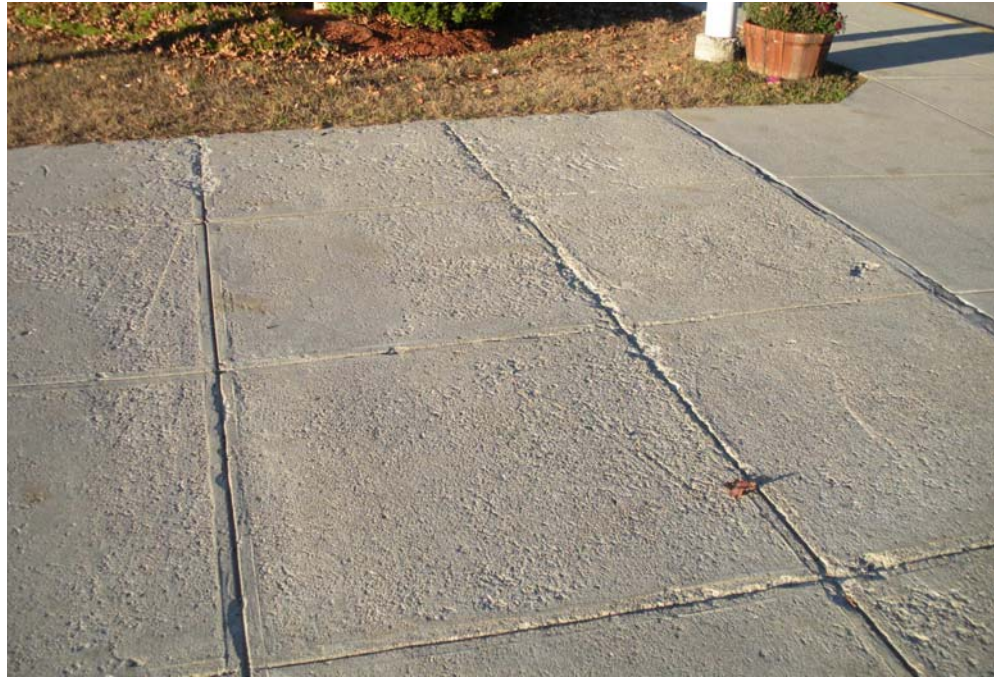
CONCRETE DETERIORATION IN PLAZA/WALKWAY NEAR FRONT ENTRANCE
