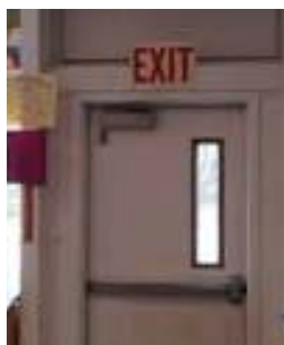
FIG 2: EXISTING EXIT SIGNS
