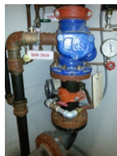
FIRE PROT. PIC 1
