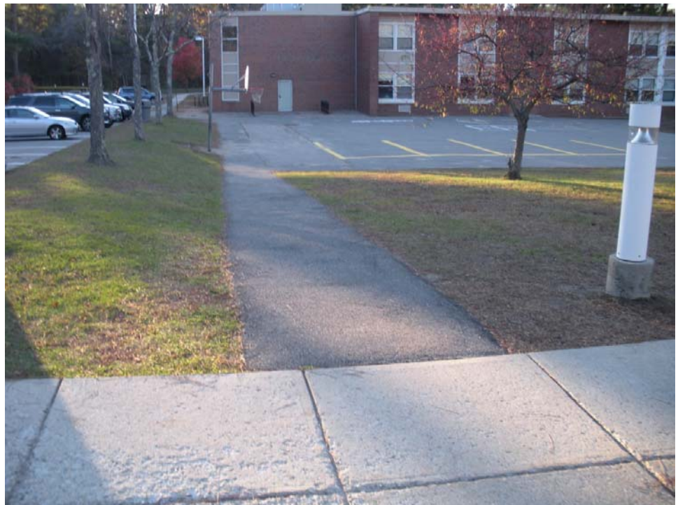
WALKWAY TO BITUMINOUS PLAY AREA/BASKETBALL COURT EXCEEDS MAAB SLOPE REQUIREMENTS
