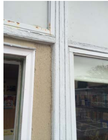
SINGLE GLAZED WINDOWS AND RUSTING STEEL FRAMES
