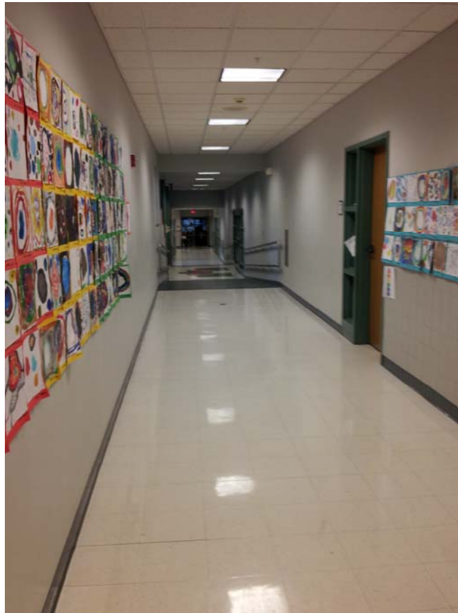
DRY ENVIRONMENT CONDITIONS CAUSE FLOOR AND CABINET PROBLEMS
