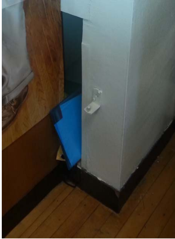
TYPICAL CLASSROOM VENTILATION EXHAUST OPENING ALMOST COMPLETELY BLOCKED BY A STORAGE CABINET.
