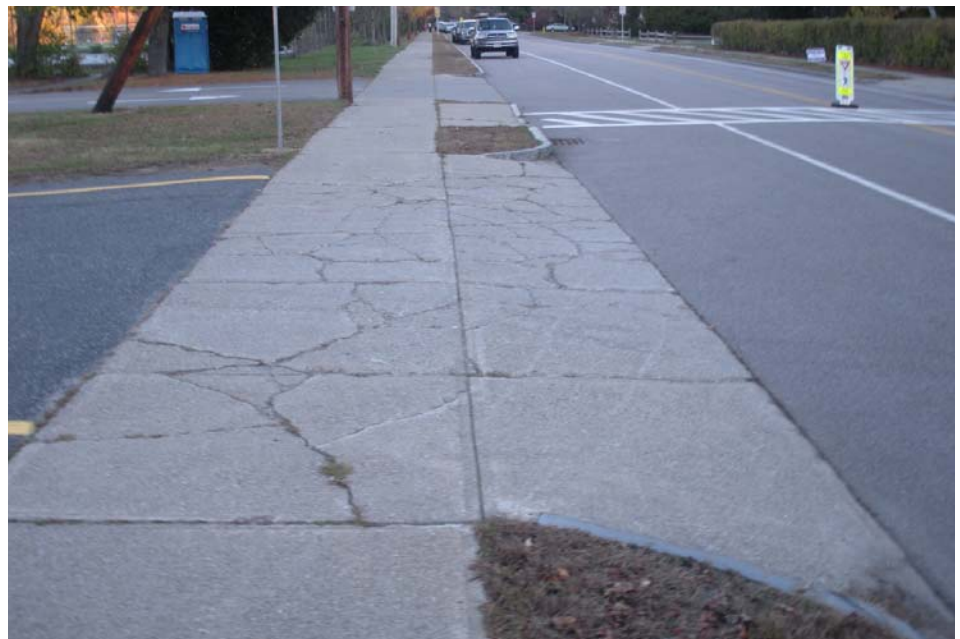
BLOCK AND FATIGUE CRACKING AT CONCRETE ENTRANCE APRONS
