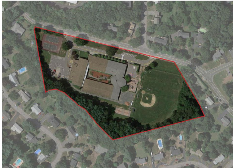
Downey Elementary Minor System Upgrades Minor Interior Fit-Up
