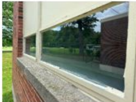
Image 16 – Deteriorated glazing, single pane (1957)
