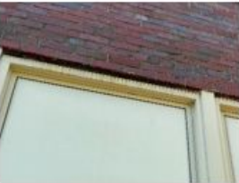
Image 14 – rusting lintels at 1939 wing
