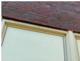
image 14 – rusting lintels at 1939 wing
