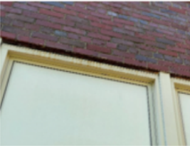
Image 14 - rusting lintels at 1939 wing
