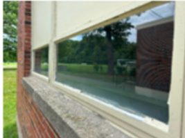
Image 16 – Deteriorated glazing, single pane (1957)
